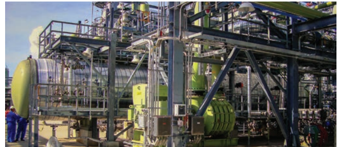
Reaction Furnace Waste Heat Boiler
