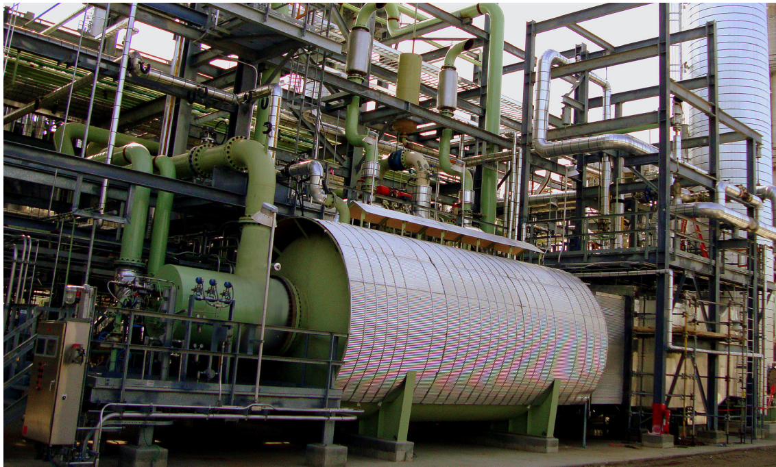
SRU Tail Gas Thermal Oxidizer with watertube style waste heat boiler
